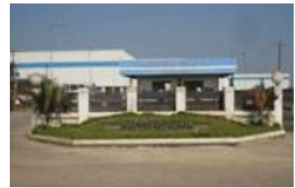
Unit 2 - Chakan, Pune, Maharashtra (Area - 58,364 sqm)
