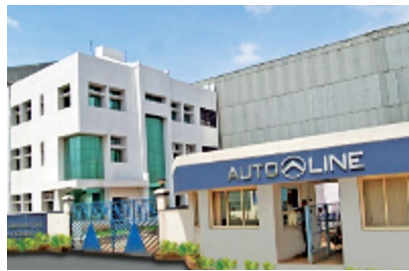
Unit 1 - Chakan, Pune, Maharashtra (Area - 11,400 sqm)
